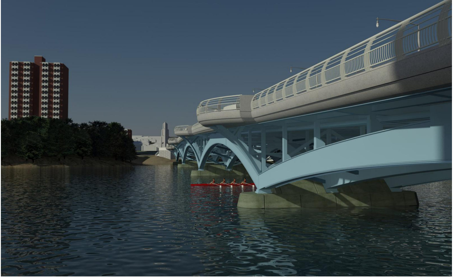
Figure 2: Rendering of the Proposed Steel Deck Arch
